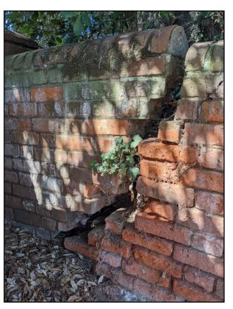
Figure 24 Damage to Brightlingsea Hall boundary wall
