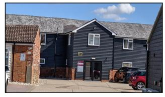
Figure 23 Loss of historic features within the barn complex can be seen with replacement windows, doors and roofing
